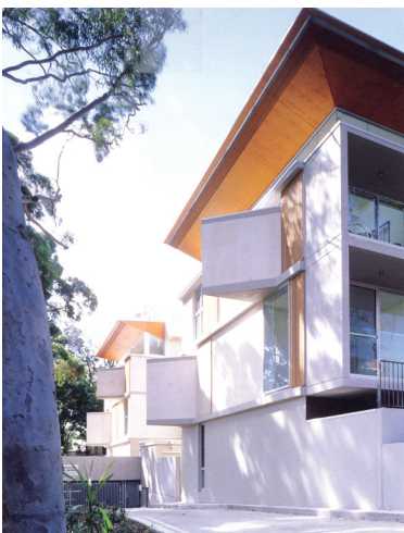
Discreet car parking entry that is well concealed from the street, optimising on the site's topographical features.
