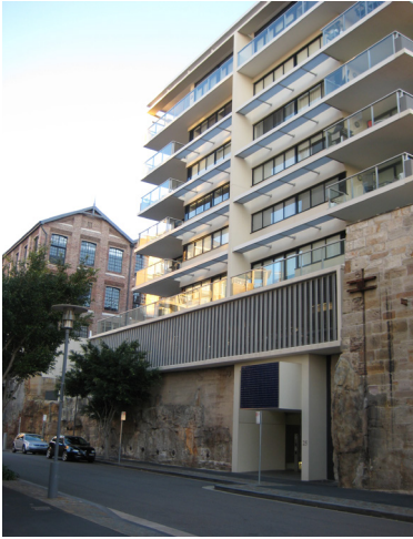
Car parking facade that is well integrated into the overall composition of the building base.
