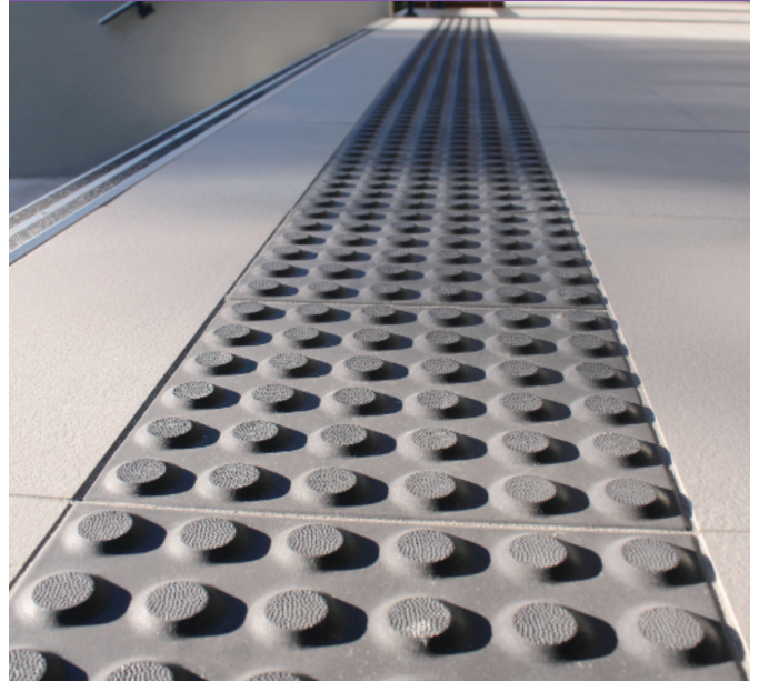
Sample - Ceramic warning tactile ground surface indicators
