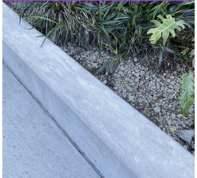
Sample - 200mm Wide insitu concrete retaining wall
