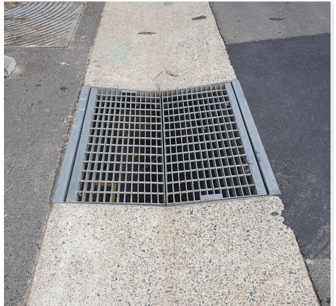
Sample - V-drain swale
