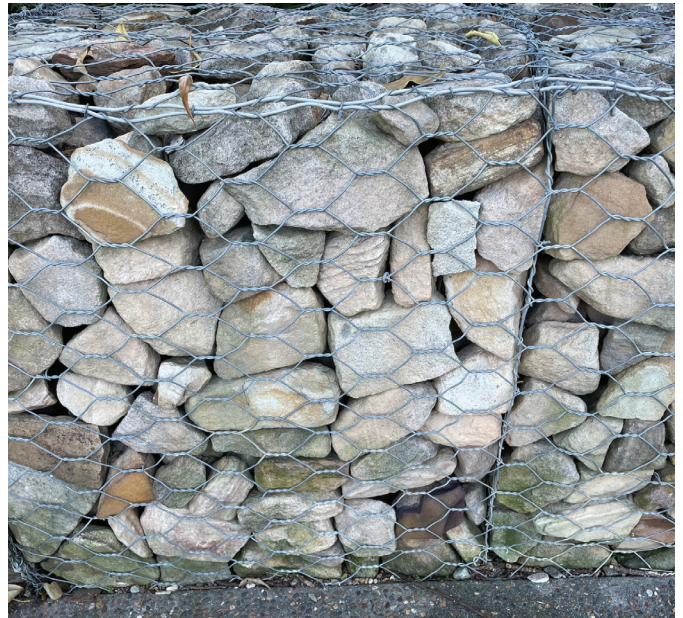
Sample - Gabion wall
