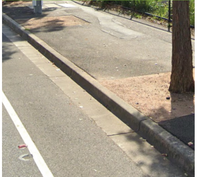
Sample - Insitu kerb & gutter - standard size
