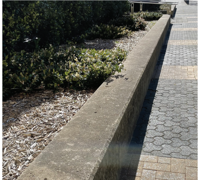
Sample - 400mm Wide Insitu concrete wall
