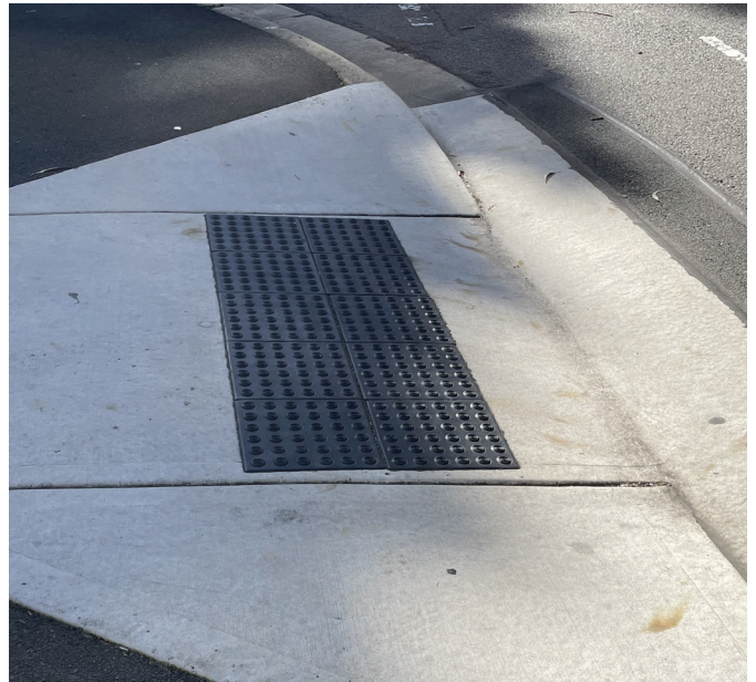
Sample - Standard kerb ramp
