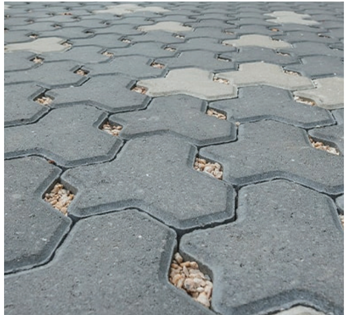
Sample - Ecotrihex 80 permeable pavement
