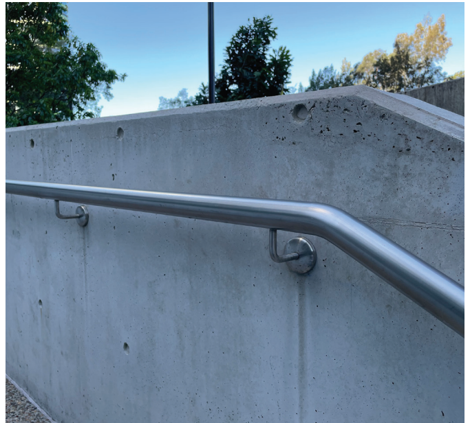
Sample - Handrail - wall mounted
