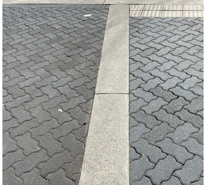
Sample - Precast flush kerb
