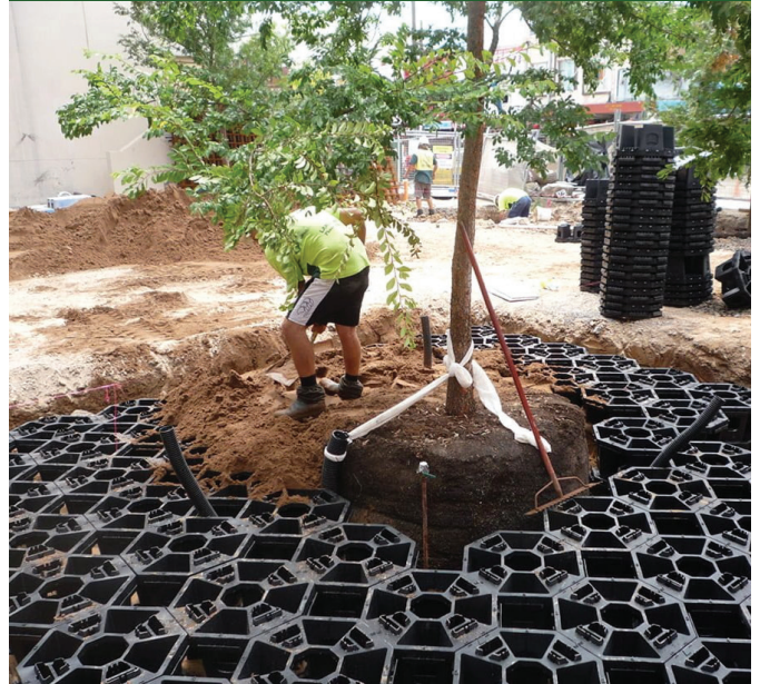
Sample - Tree planting with soil vault system
